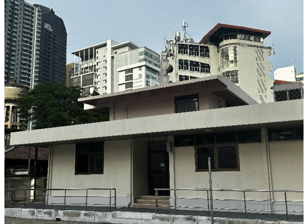
Photo 21 - Second Floor added in 1976.
