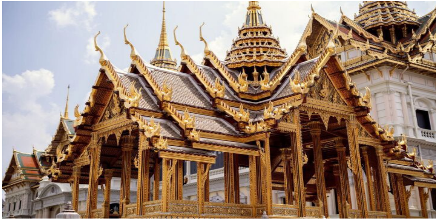
Photo 8: A portion of one of the structures at the Royal Palace in Bangkok
